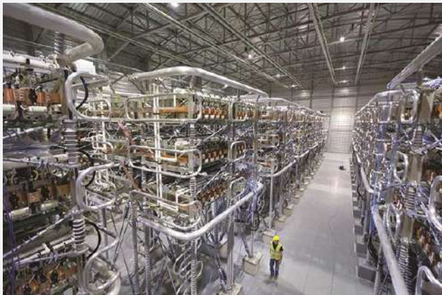
Figure 1. HVDC converter station, Source: "Benefits of High-Voltage Direct Current Transmission Systems", https://www.powermag.com/benefits-of-high-voltage-direct-current-transmission-systems/
