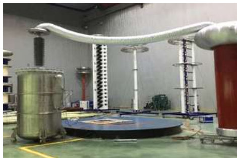
Figure 7. Partial discharge test site
